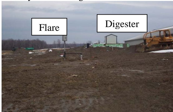
Digester and Biogas Flare
