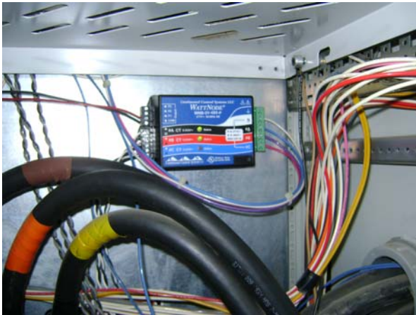
WattNode Power Transducer (WG1)
