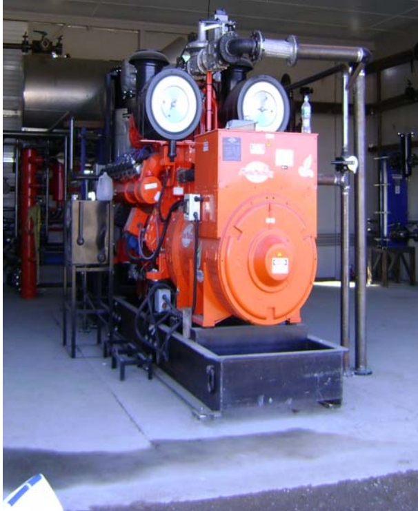
Partially Installed Engine Skid
