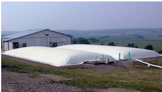
Covered Digester and Support Building
