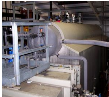
Typical heat recovery steam generator
