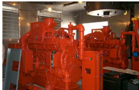
Engine-Generator Sets During Installation
