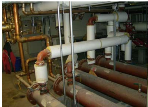
Typical DHW Heat Exchanger Network
