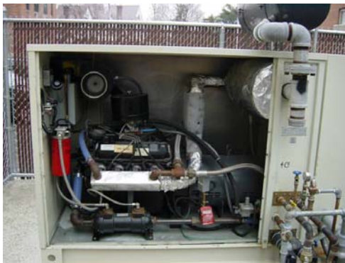
Typical Engine Heat Recovery Piping
